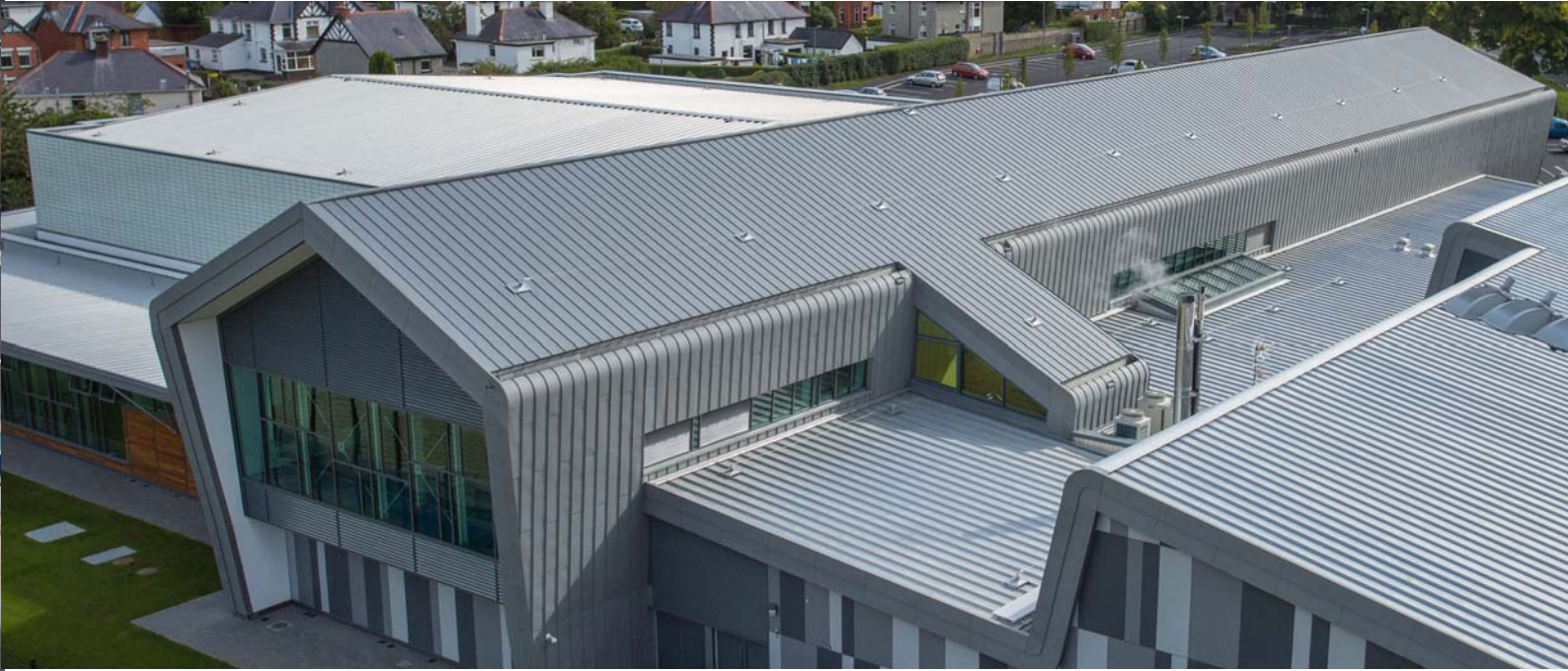
Typical APL non-combustible ZipSeam™ standing seam assembly
